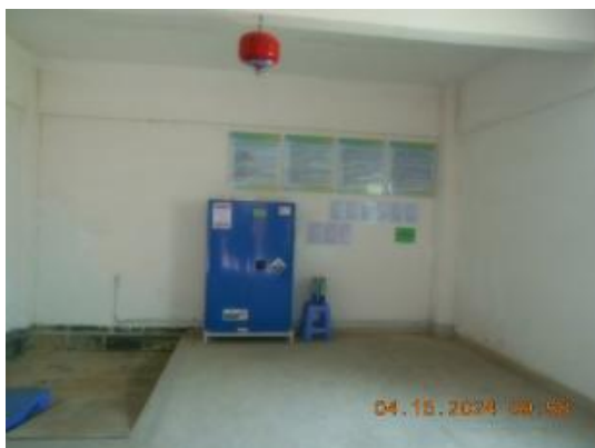
Hazardous chemical warehouse.JPG
