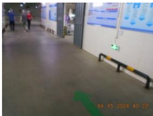
Main aisle with evacuation sign.JPG
